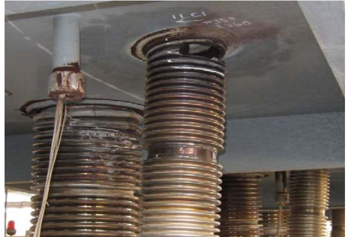
Typical metal bellows fatigue failure due to frequent HRSG shut downs
