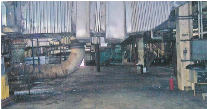
Original metal box-fold expansion joint lagged with insulation
