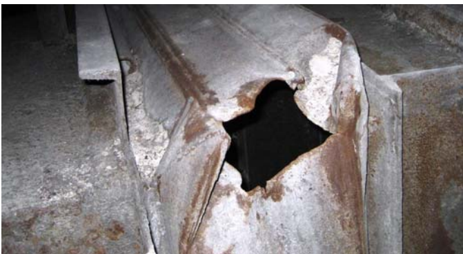
Single and double-mitered, and camera corner designs often tear at the welds
