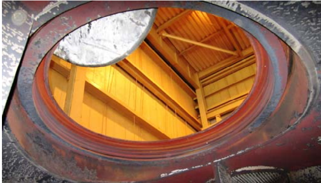
View from inside the LP turbine with cross-over pipe removed
