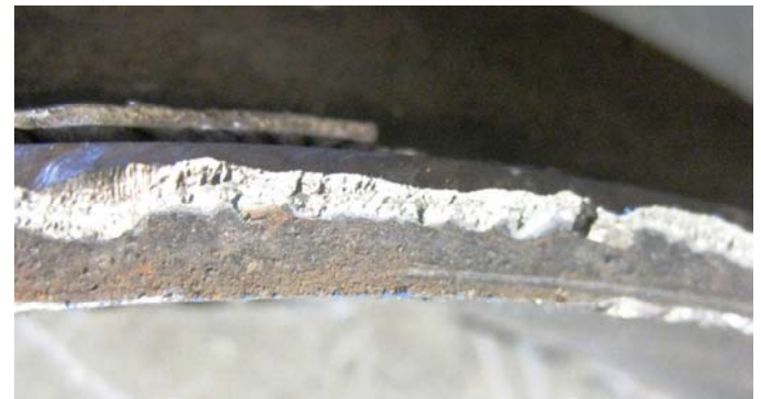
This failed liner attachment weld had very little penetration
