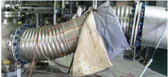
Unsupported pressure thrust extends expansion joint metal bellows
