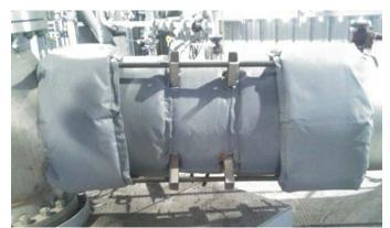
Newly installed limits rods are added insurance
